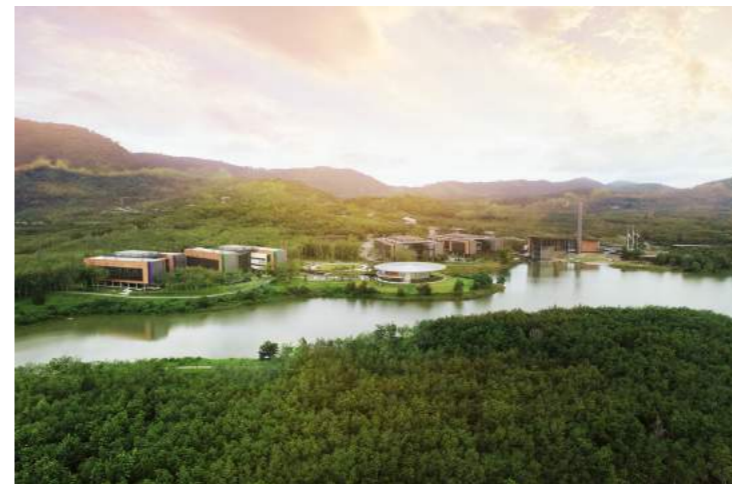
2015 VIDYASIRIMEDHI INSTITUTE OF SCIENCE AND TECHNOLOGY (VISTEC) Wang Chan Valley, Rayong
